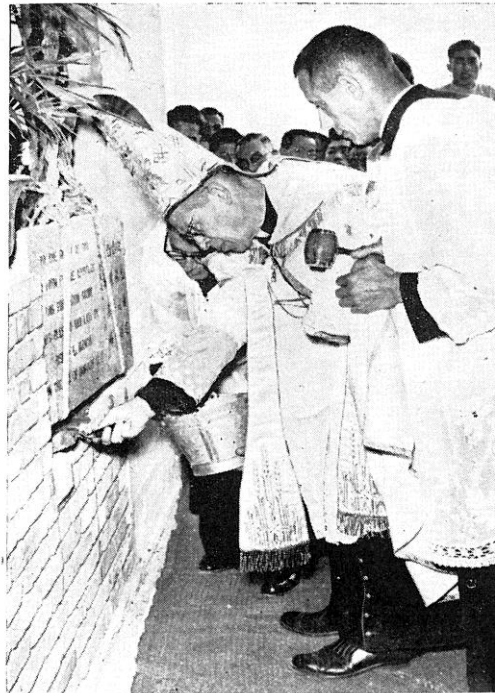
The Stone is Laid
