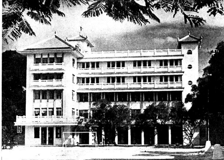
The new wing at Holy Spirit Seminary, Aberdeen, Hong Kong.
