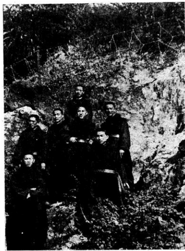
Some of the young Trappist monks on the site of the new Monastery at Lantao Island. Eleven are on the island at present preparing the soil for planting, and making tracks from the wharf to carry the materials for the building to the site.
